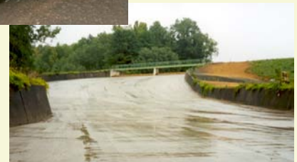
Dam Spillway After Repairs
